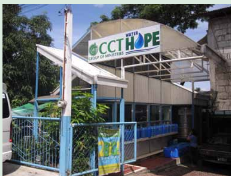
A WaterHope community water station in the Philippines.
